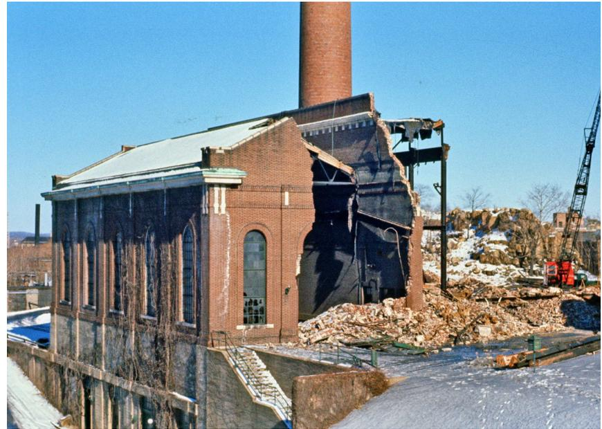
During demolition, a decommissioned WWII tank was used to pull down the plant chimney. Courtesy of Thom Cronin.
