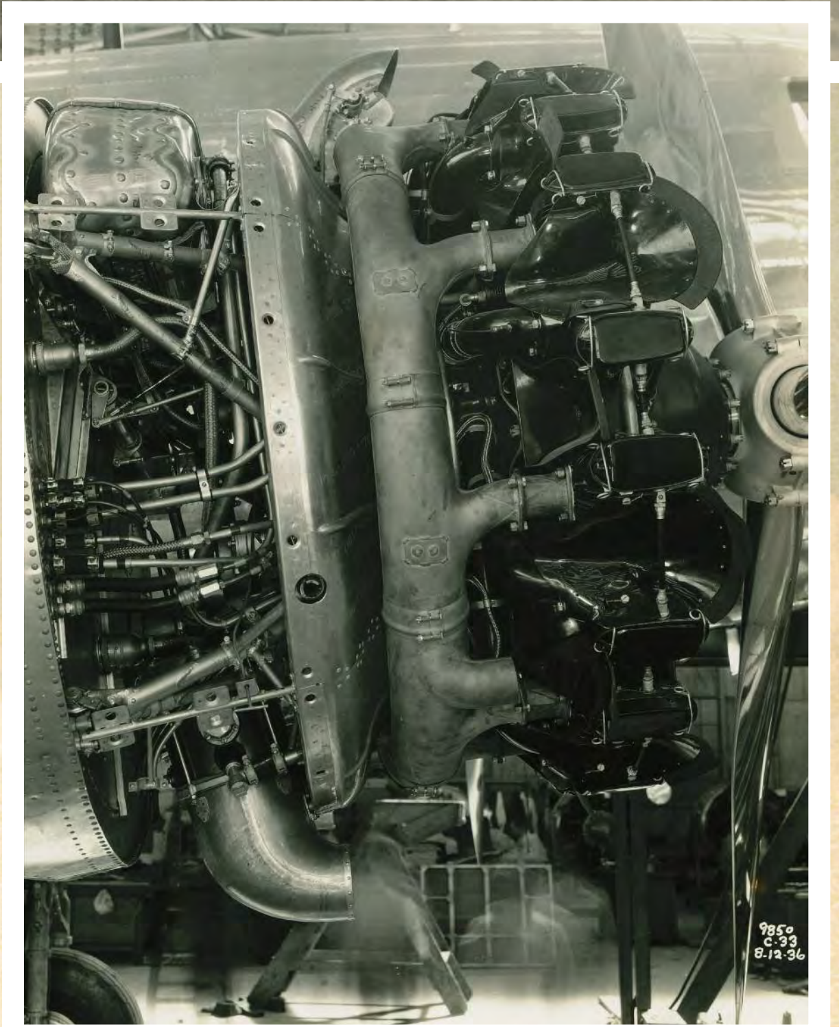
Wright R-1820 Cyclone engine used in Douglas DC-2 C-33.
