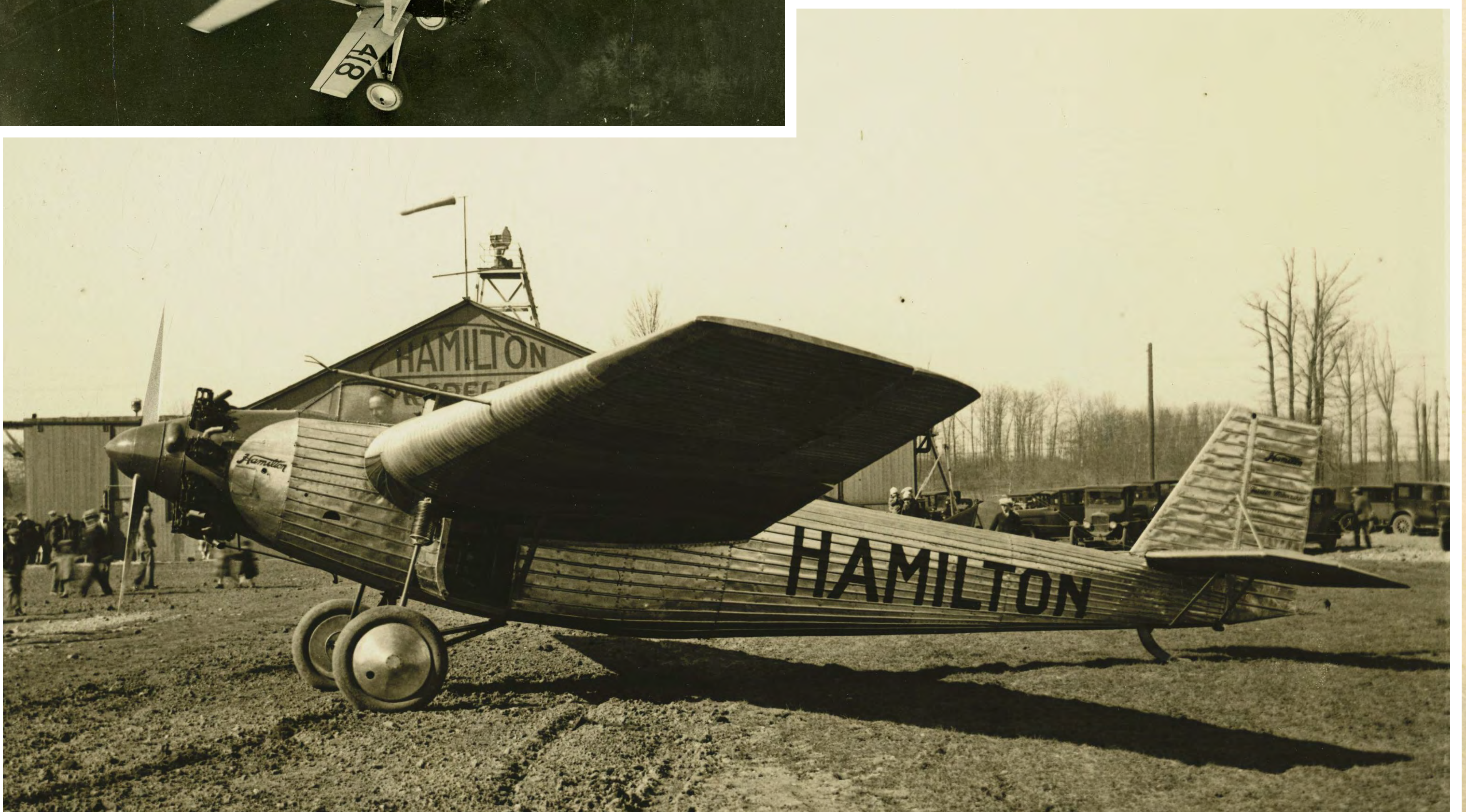
Hamilton H-47 Special, powered by a 525 hp Wright Cyclone engine. The only one of its kind, 1928.
